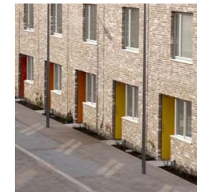
5. Full timber, painted front doors with glazed sidelight in differing colours along the street.
